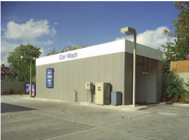
This wash housing is constructed of COMPOSOLITE® 3-way connectors, toggles and panels. No internal structure is required. Dimensions are 36' x 16' x 14'-3/4" high. Low maintenance, ease of construction and an attractive appearance were the benefits to the customer.
