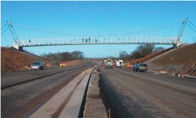
The Wilcott pedestrian bridge, in Shropshire, England, was constructed from COMPOSOLITE® panels, 3-way connectors and toggles. The bridge, which is 163' long and more than 7' wide, was built in three units and spliced to fabricate the total length.
