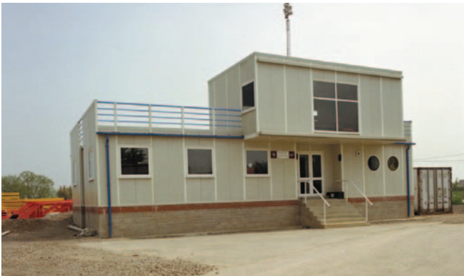
A visitor center in Bristol, UK, is constructed of COMPOSOLITE® panels, 3-way connectors and toggles with no supporting frame. Cells of panels and 3-way connectors were filled with foam for thermal insulation.
